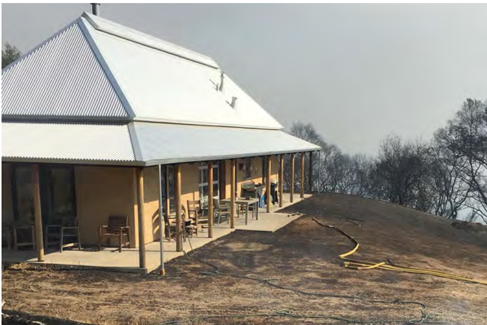
Photo – Ed Doody, taken the morning after it survived a wildfire. This Redwood Valley home, designed by Arkin-Tilt Architects, illustrates several basic principles of resilient green building: steel roof, wide porches, and generous overhangs. The primary wall material - straw bales - has low carbon impact, and its heating and cooling costs are low. It survived the October 2017 fires while many of its neighbors did not. Proper landscape management also contributed to its survival.
